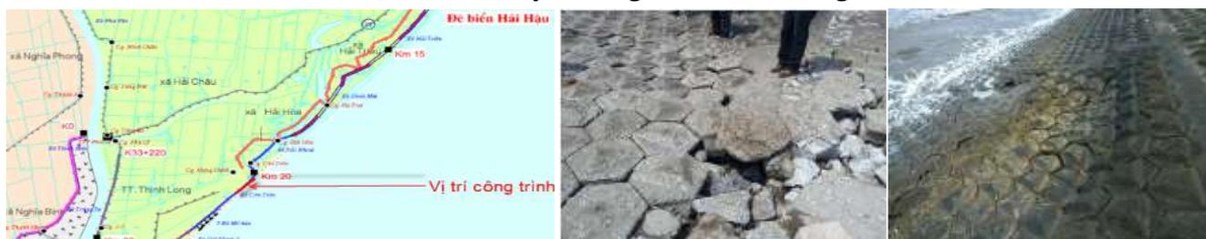
Picture 4.1- Location of the sea dyke studied      Picture 4.2- Status of sea dyke damage [10]
