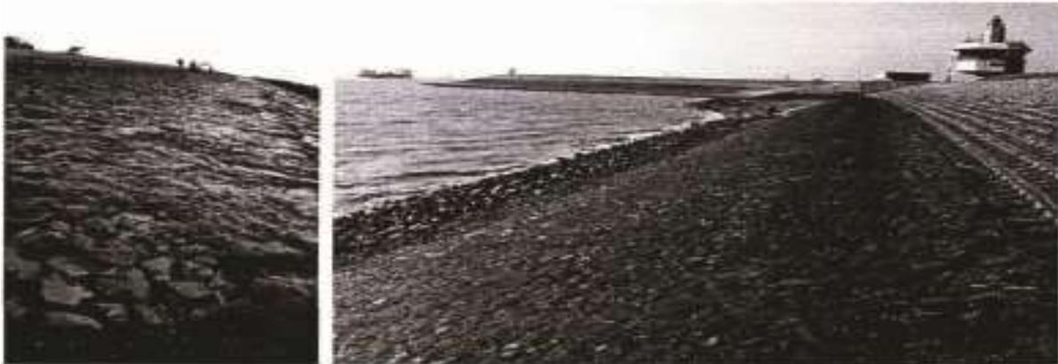
Figure 1.7- Southwest Netherlands' seawall using asphalt mortar to insert basalt [33]
