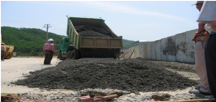
Picture 4.4. Trucking and pouring RCC
