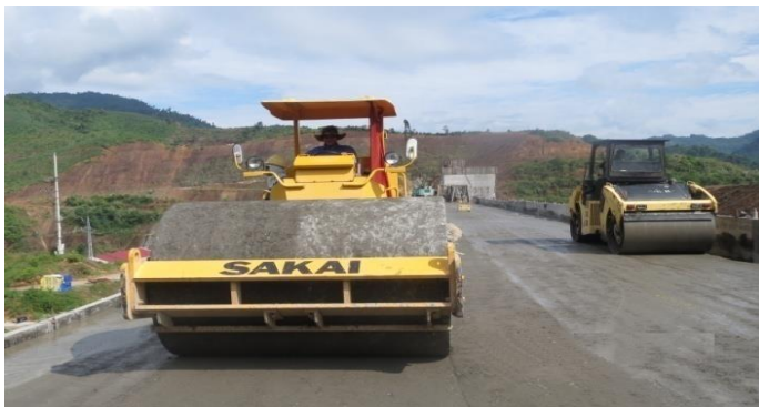
Picture 4.5. Compacting RCC
